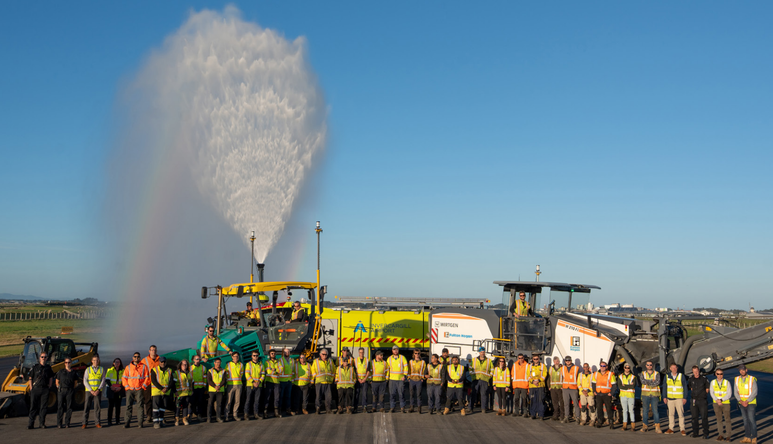
Fulton Hogan and Invercargill Airport team celebrate commencement of the final shift of runway resurfacing.
